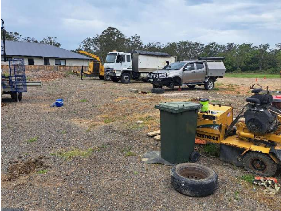
Photograph 1 – Southern Fill mound facing Southeast.
