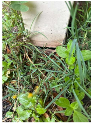
Broken down pipe base
