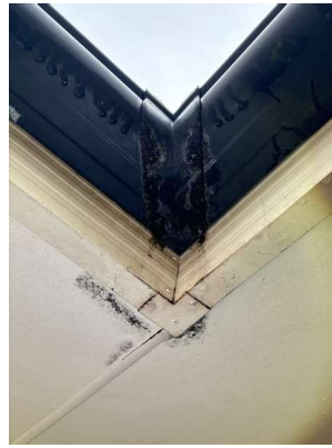
Leaking gutters
