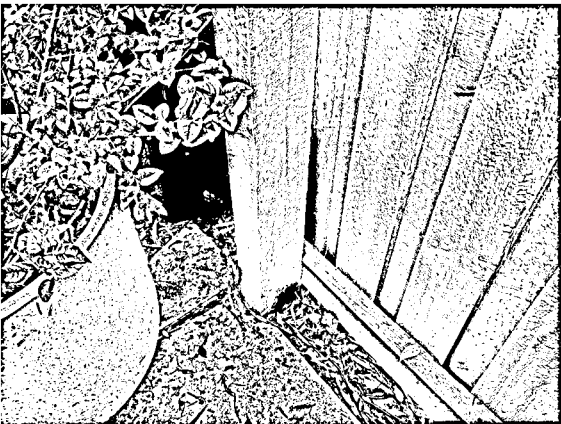
Example of surrounding timber fencing in ground contact.
